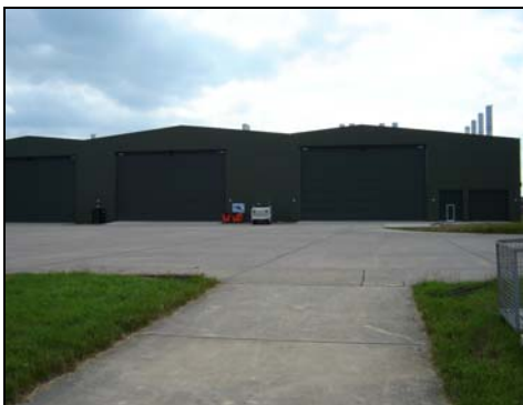
New Surface Finishing Facility
