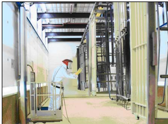
Production line spraybooth at Marshall Vehicle Engineering
